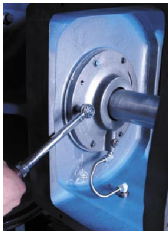
FIGURE 5-7 INSTALLING SEAL HOUSING & TUBING
