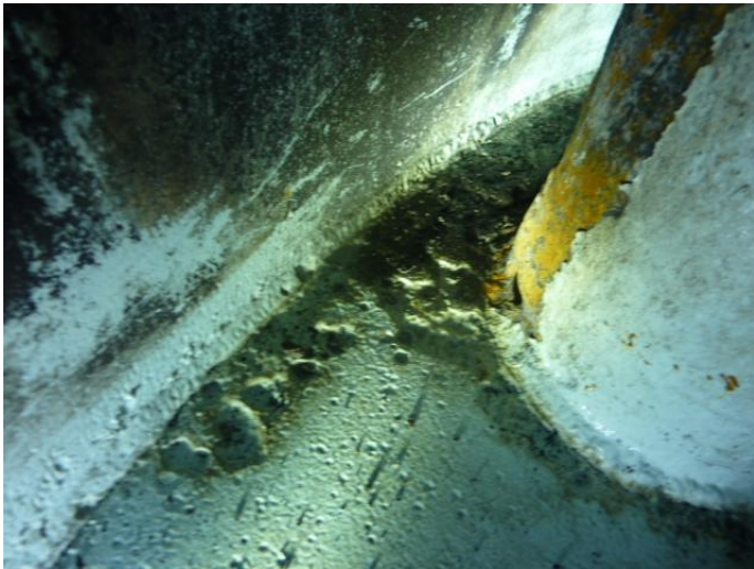
Firetube baffle corrosion
